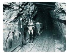
Photograph showing the removal of ore using a horse to pull a train of wagons loaded with salt and potash. Alsace, France. <u>http://www.geowiki.fr/index.php?title=Les</u> <u>Mines\_de\_Potasse\_d'Alsace\_au\_fil\_du\_temps</u>
