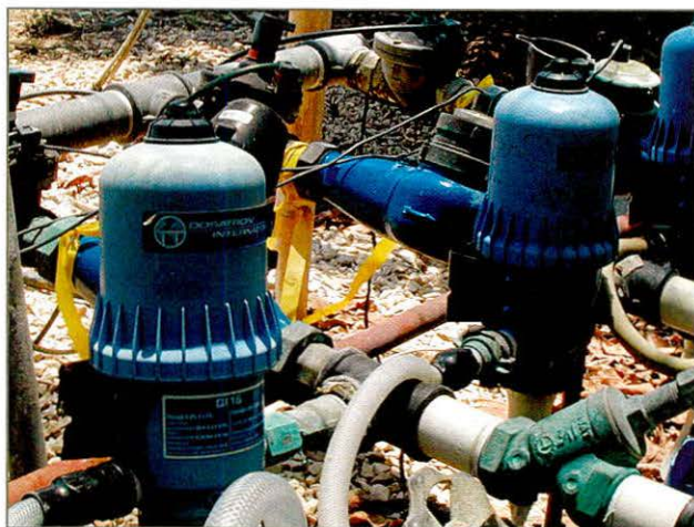
Plate 5.11. Dosatron fertilizer pump.
