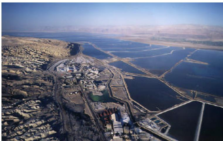
**Plate 1.2.** Potash production from solar evaporation ponds at the Dead Sea (photo courtesy DSW).
